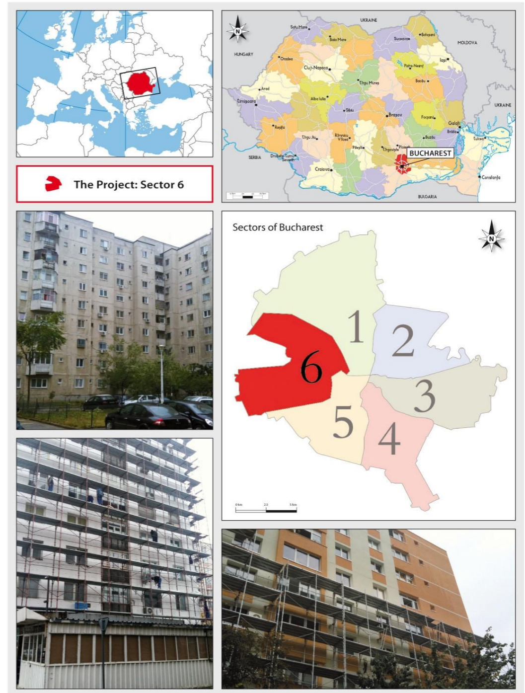
Project: BUCHAREST S6 THERMAL REHABILITATION - Romania
